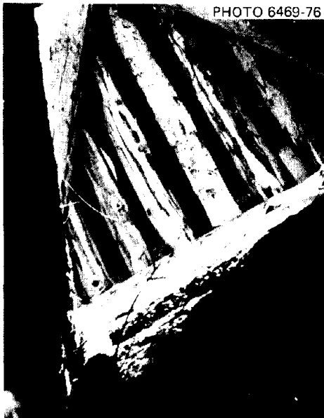
Fig. 11.6. Undamaged triangular blast door, partly open, and viewed looking up the side of the triangular entry to which the door was hinged.
